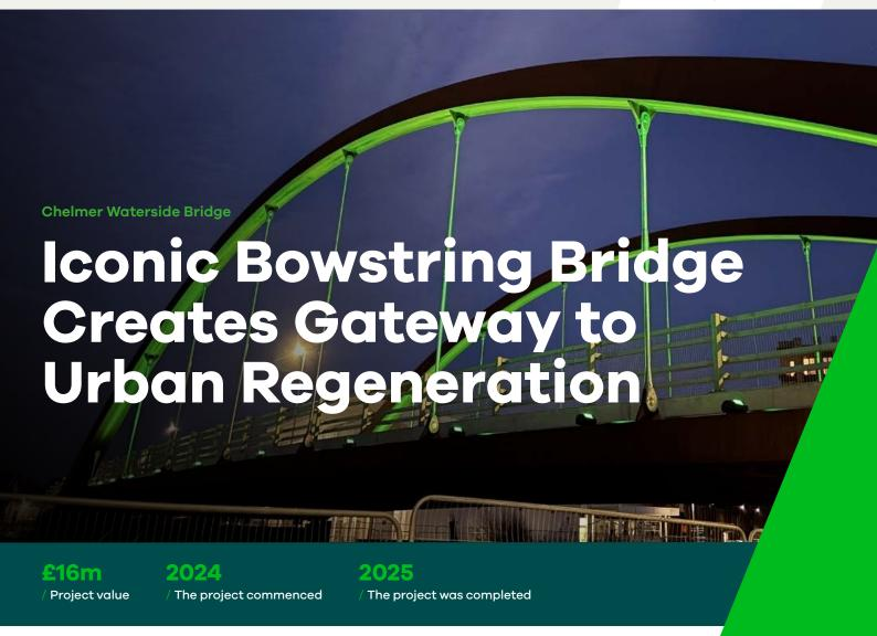
GRAHAM successfully delivered the iconic £16m Chelmer Waterside Bridge (known as "Bow Bridge Road") in Chelmsford, featuring distinctive twin bowstring arches made from weathering steel. The 50-metre pedestrian and road bridge provides essential access from Parkway to Chelmer Waterside, the city's largest brownfield site, whilst allowing for future boat navigation on the River Chelmer and supporting the area's regeneration plans, serving as a gateway to the Waterside neighbourhood.
