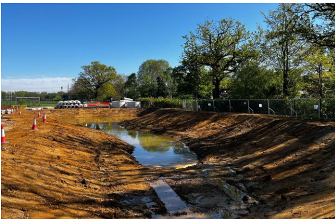
Picture 3: New Drainage Pond at Holloway Hill
