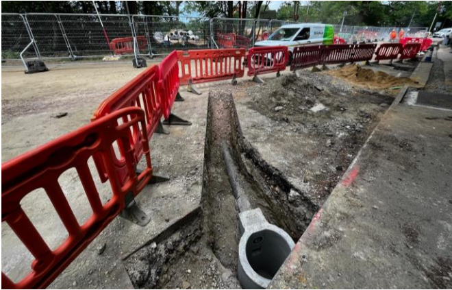
Picture 2: Installing Drainage Chambers at Holloway Hill
