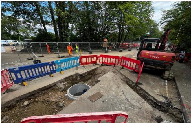
Picture 2: Installing Drainage Chambers at Holloway Hill
